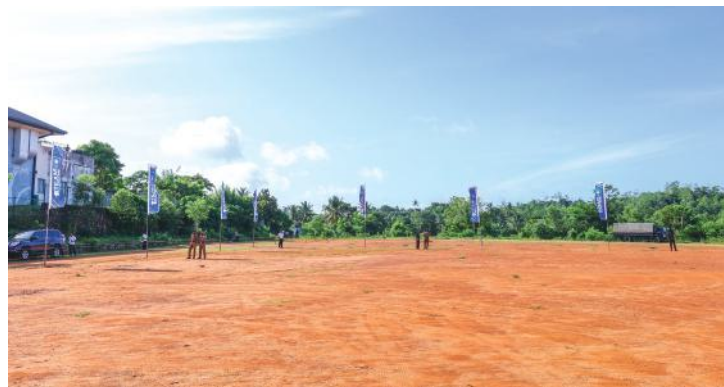
The cricket ground being readied for construction.
